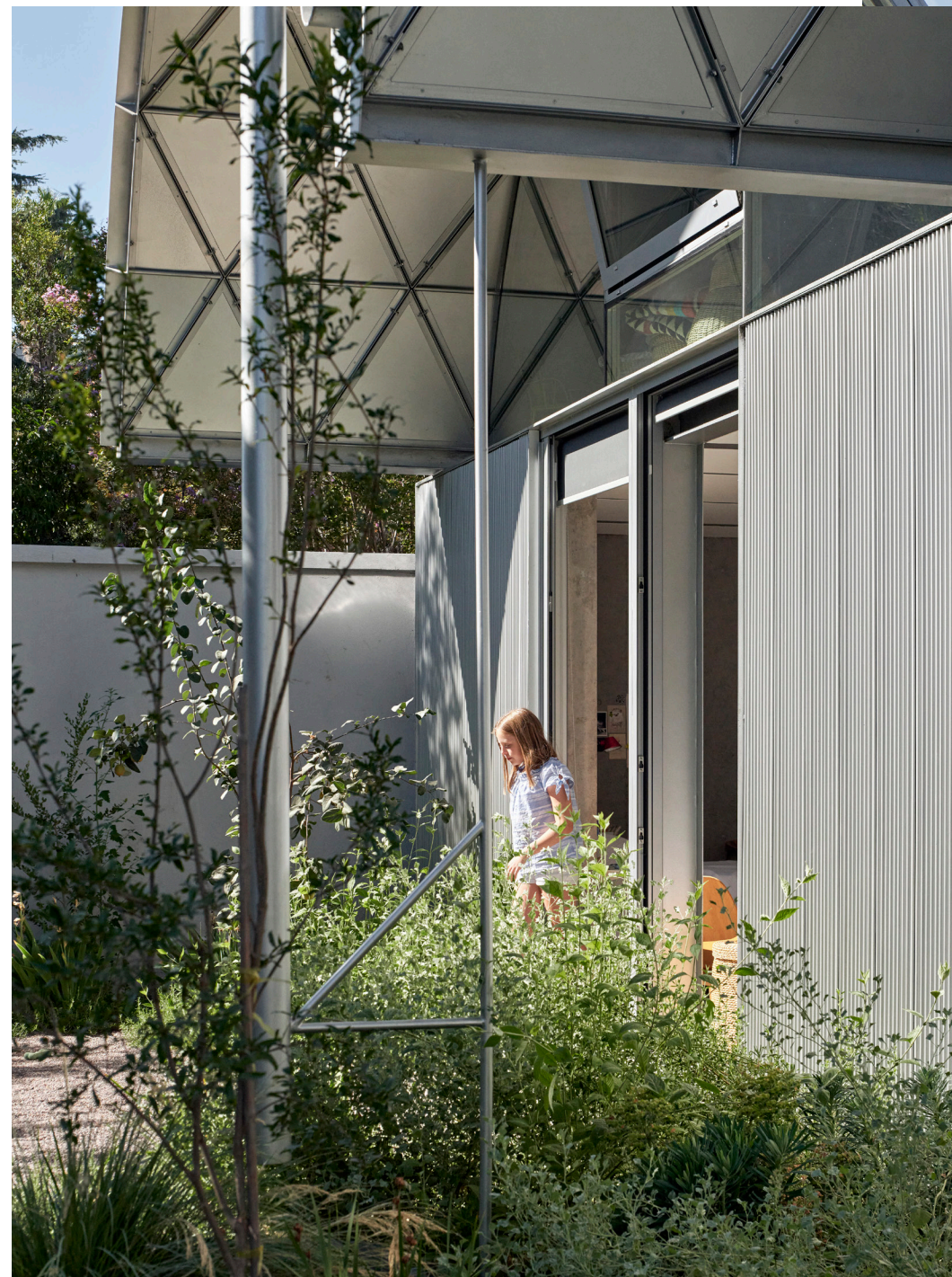
The kids’ room (above) has two doorways so it could be split. Emilia had concerns about the coolness of her husband’s design. “I’m the kind of person who likes Victorian cottages,” she admits. “But if you look at the details of the steel and how the structure is
